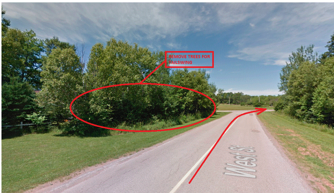
West Road to East Royalty Road- Tree Removal
